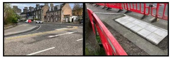
At Links Place we are installing new tactiles and also a new central pedestrian island, please see below for further details on the westbound bus gate that will be implemented here.
